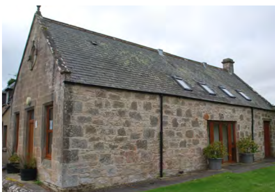
Figure 11. Lethen Road Hall, Auldearn
