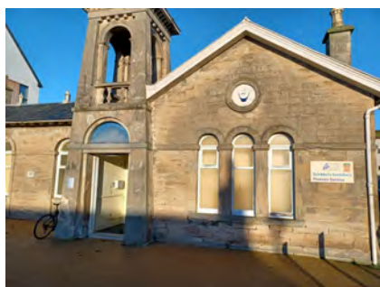
Figure 9. Italianate School Building
